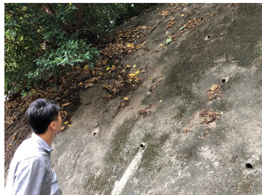
(4)楠興宮旁護坡擋土噴漿
