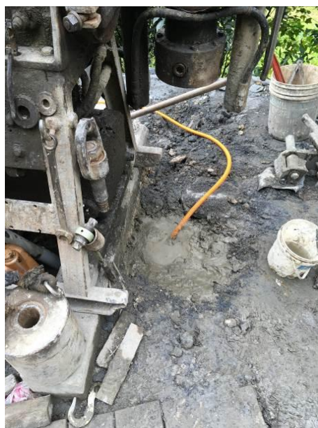
Figure 4.1.2-6 In-situ installation of TDR deformation monitoring cable in 108-D007-2T
