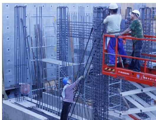
(c) 組裝對角向鋼筋
