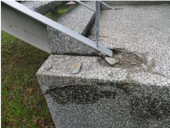
(a)東側戶外樓梯
