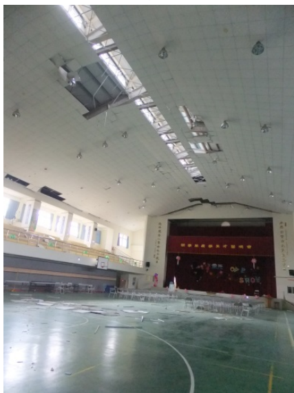
(a)館場天花板全貌
