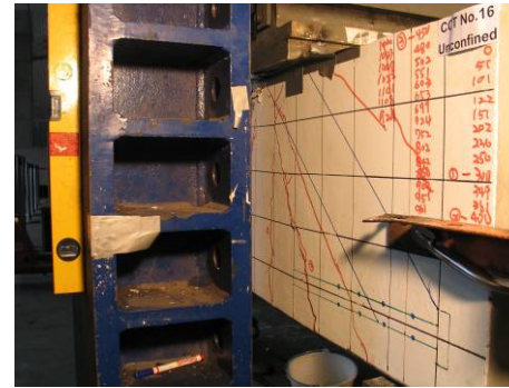
(k) Failure Point
