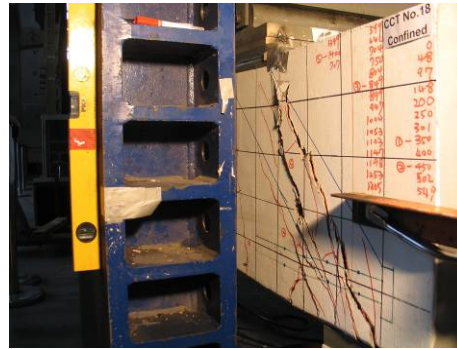
(j) Failure Point
