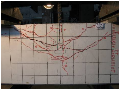
(p) Failure Point
